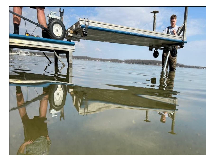
Figure 17: Installing a Dock Section
